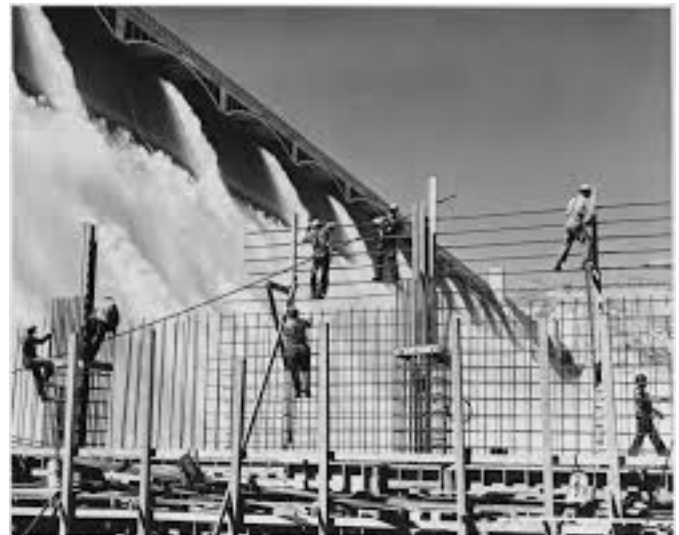
FIGURE 1: GrandCoulee Dam Under Construction
